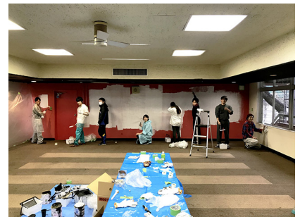
Students painting the facility walls...
