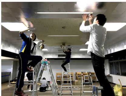
Renovating the ceiling...
