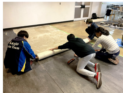
Installing new flooring...
